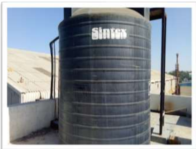
Overhead Storage tank for RO Rejected water
