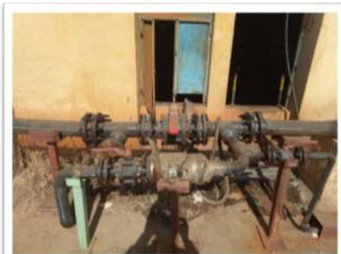
Auto Control Valve Station
